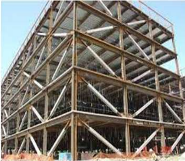
Fig 2.7 Buckling Restrained Brace
